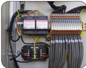
Dataline with the Strikesorb DRM Modules
